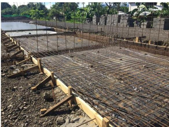
Image showing reinforcement placement for the outer office floorslab.
