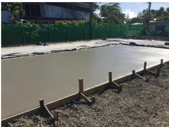
Image of the completed concrete pour for the warehouse slab.
