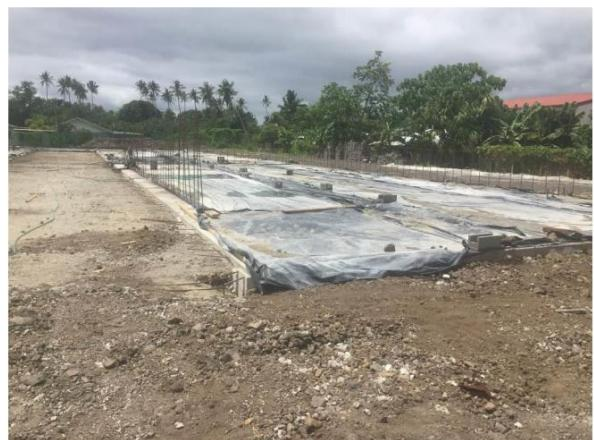
Image showing completed concrete works for the floor slabs. A small portion is left in the middle to allow for the crane to maneuver in place when erecting the structural steel.
