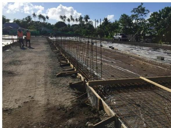
Image showing reinforcement placement for the inner office floor slab and intermediate strip footing for the internal block wall.
