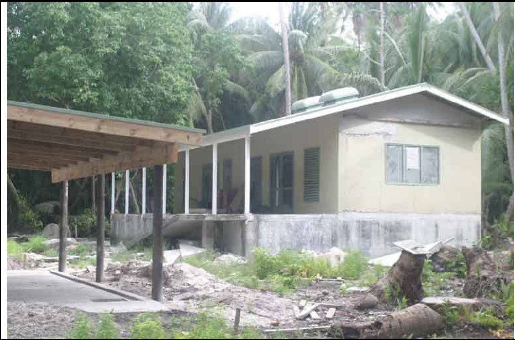
Figure 2-3 – New Power Station on Fakaofu
